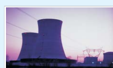
Thermal power station
