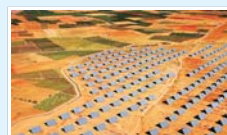
Solar power station
