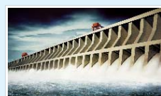
Hydraulic power station
