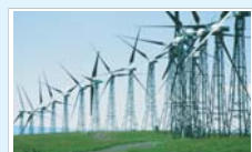
Wind Power station
