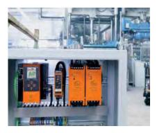
Gateways allow connection of AS-i to different fieldbuses.
